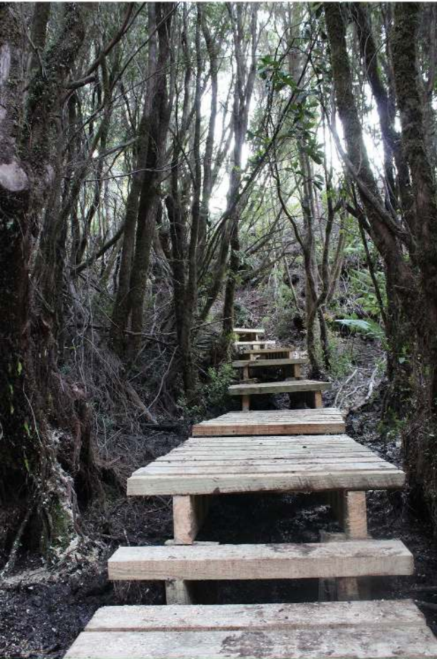
ECOLOGICAL TRAILS - In 2017 we began the construction of our Nature Discovery Center, located in the Valdivian rainforest.
